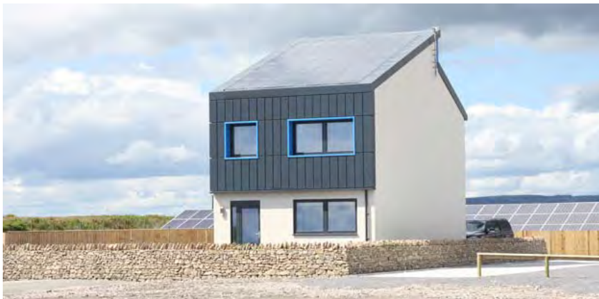
SOLCER house. Source: Cardiff University
